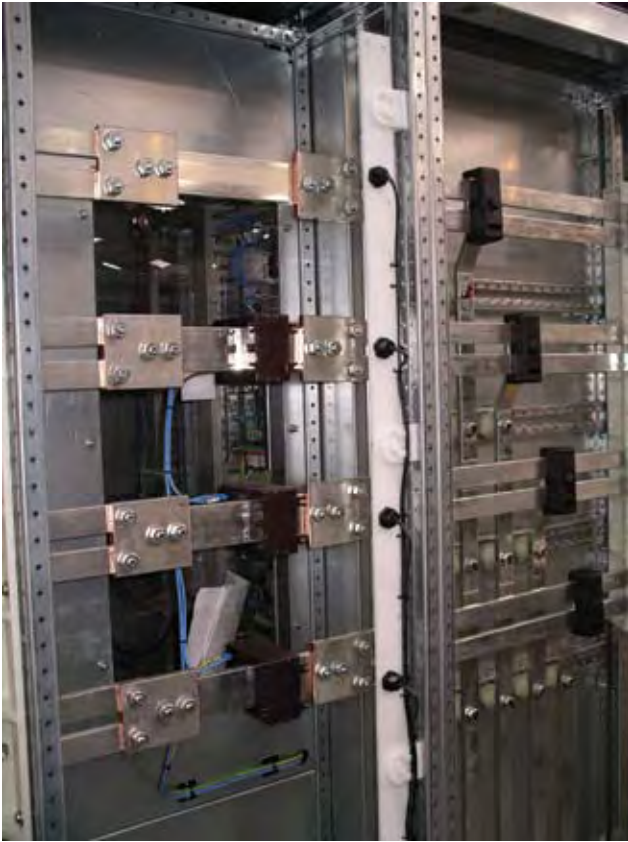
Figure 2 - Unobtrusive installation and the convenience of no maintenance make constant thermal monitoring an attractive option for critical equipment.
